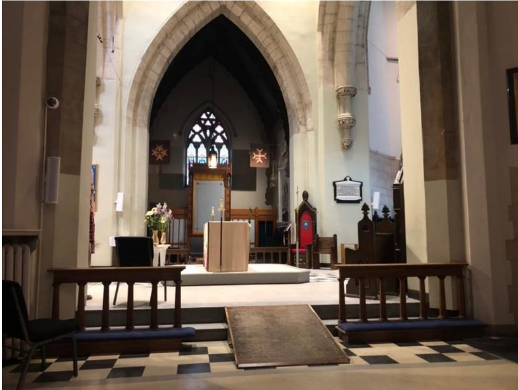
Illustration 22 - Removable wooden railing on the right side of the transept
