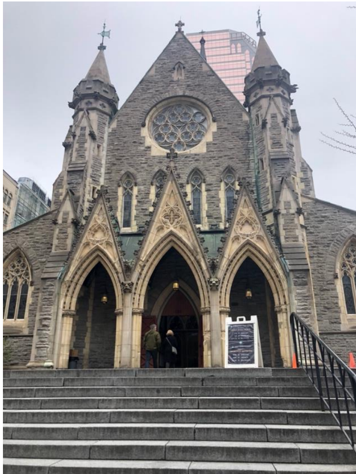
Illustration 17 - View of the cathedral from the bottom of the steps
