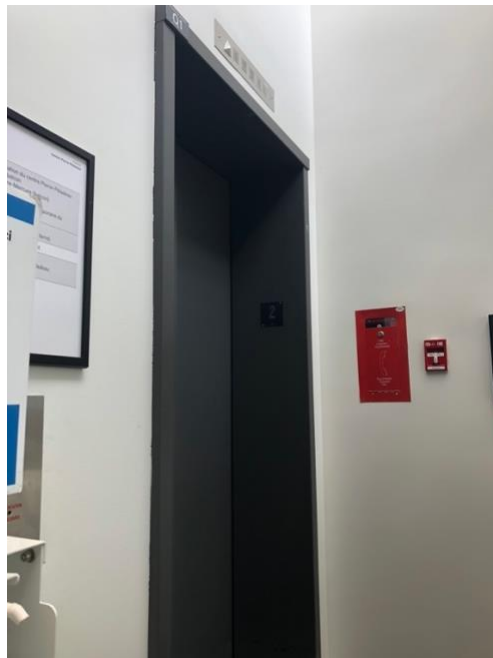
Illustration 10 - Elevator on the street side
