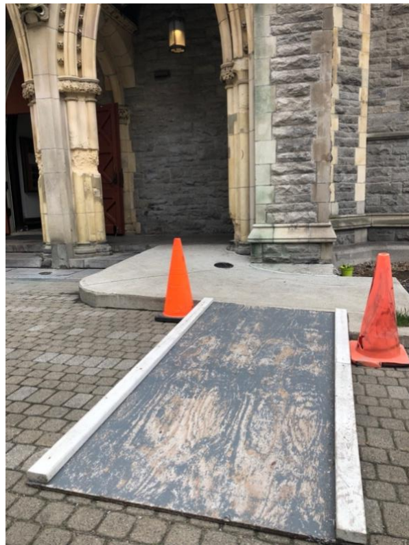
Illustration 20 - Access ramp to the church
